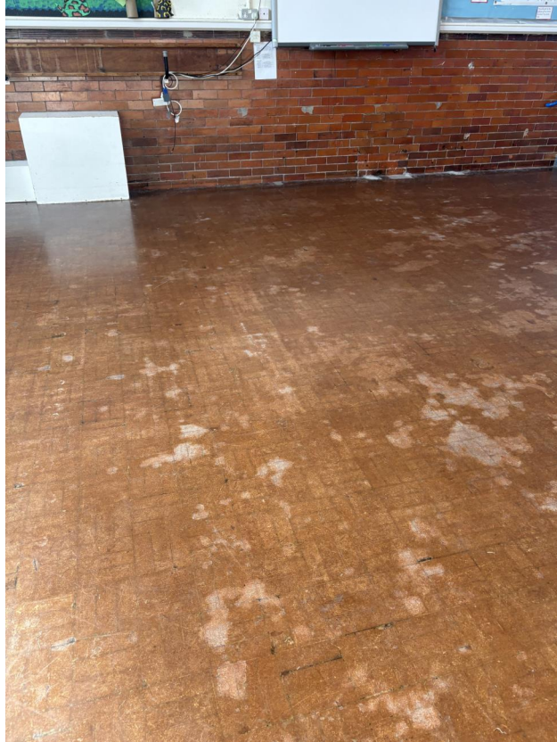
3 - Hall floor before
